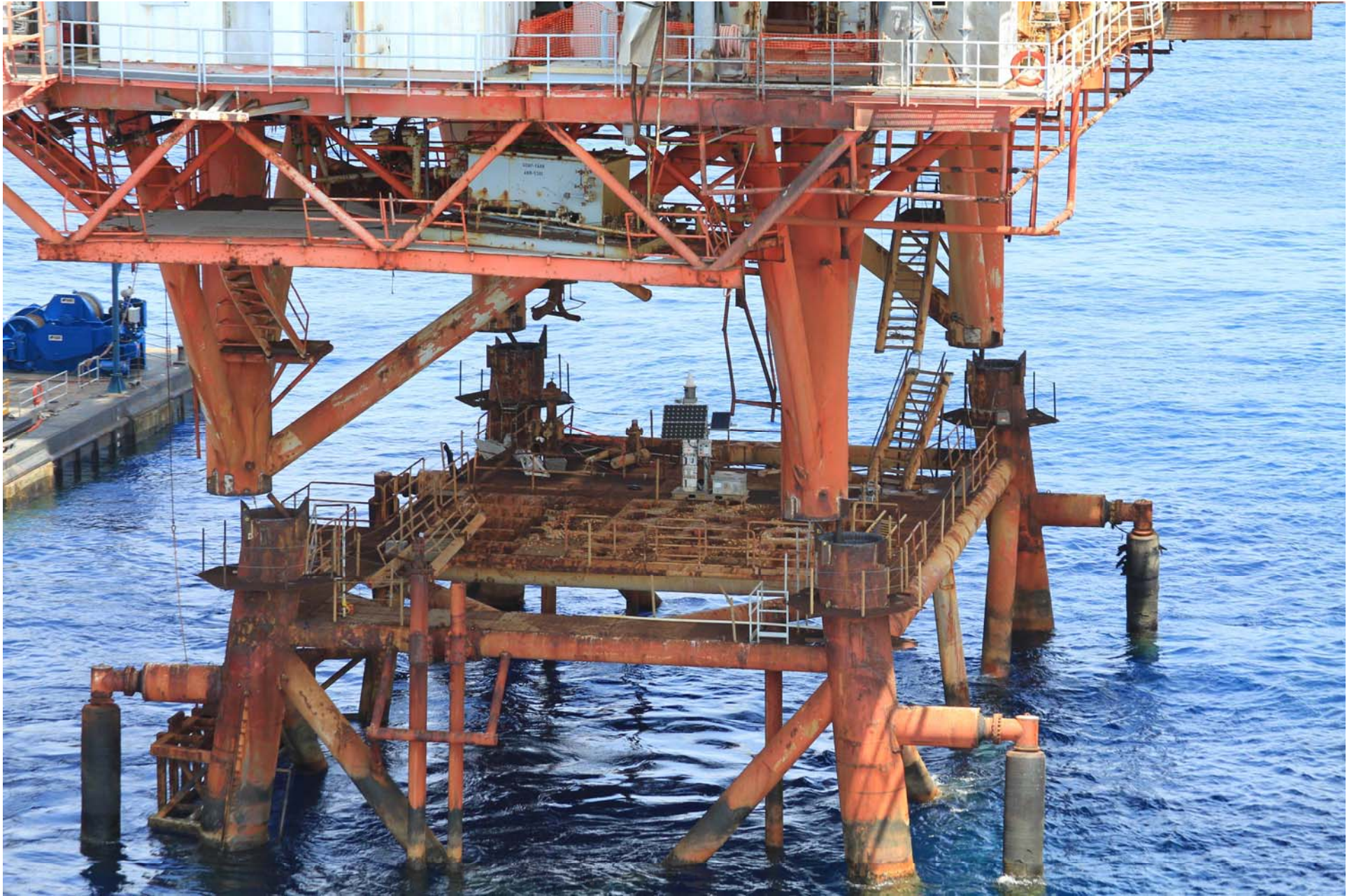
As soon as the topside is free of the jacket, the VB – 10000 begins to maneuver clear.
